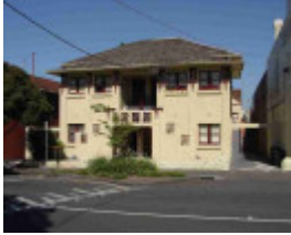
richmond lennox street richmond lennox street 176- 178 unit 1-10
