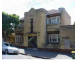
carlton north pigdon street carlton north pigdon street 146
