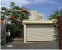
richmond brock place richmond brock place 15
