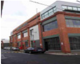
cremorne balmain street cremorne balmain street 64 unit 13
