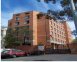
Richmond Church Street 353-355 rear.JPG
