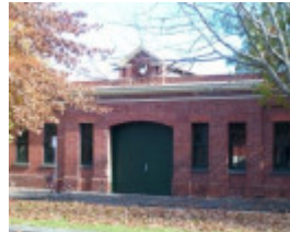
Cable Tram Engine House
