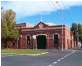
Cable Tram Engine House
