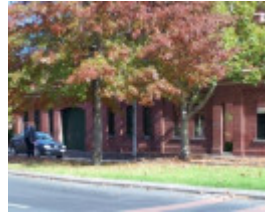
Cable Tram Engine House
