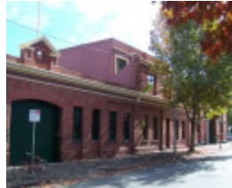
Cable Tram Engine House
