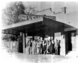
207 - JN Burgoyne 820 Main Rd Eltham 03 - This shop photographed after the south side addition was completed (ELHPC No. 702) - Shire of Eltham Heritage Study 1992
