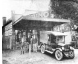
207 - JN Burgoyne 820 Main Rd Eltham 02 - J.N. Burgoyne's shop as built - Note the exterior and its details (ELHPC No. 701?) - Shire of Eltham Heritage Study 1992
