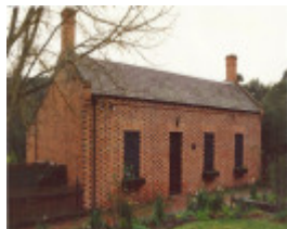
Shillinglaw Cottage Main Rd Eltham Colour 2 - Shire of Eltham Heritage Study 1992
