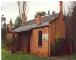
Shillinglaw Cottage Main Rd Eltham Colour 3 - Shire of Eltham Heritage Study 1992
