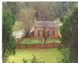
Shillinglaw Cottage Main Rd Eltham Colour 1 - Shire of Eltham Heritage Study 1992
