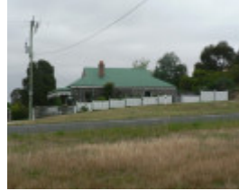
Athelston, 2025 Hamilton Highway, Murgheboluc viewed from north.
