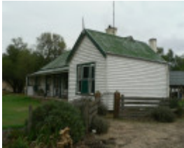
Former Harvey Farmhouse, 2000 Hamilton Highway, Murgheboluc
