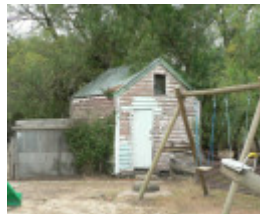
Former Harvey Farmhouse, 2000 Hamilton Highway, Murgheboluc
