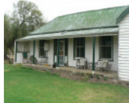
Former Harvey Farmhouse, 2000 Hamilton Highway, Murgheboluc
