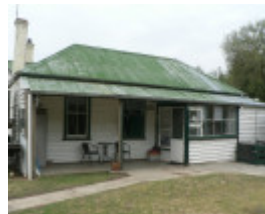
Former Harvey Farmhouse, 2000 Hamilton Highway, Murgheboluc
