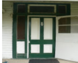
Former Harvey Farmhouse, 2000 Hamilton Highway, Murgheboluc
