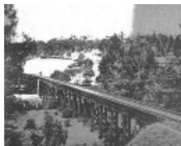
Railway Timber Trestle Bridge, Panther Place - OLD PHOTOGRAPH
