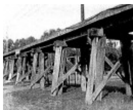
Railway Timber Trestle Bridge, Panther Place
