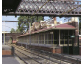
1 railway station complex ferrars street south melbourne trackside view feb1999
