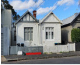
16 - 17 Mell Street Toorak
