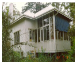
Stanhope House Eltham Colour 3 - Shire of Eltham Heritage Study 1992
