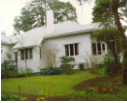
Stanhope House Eltham Colour 4 - Shire of Eltham Heritage Study 1992
