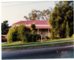
House 123 Pitt St Eltham Colour - Shire of Eltham Heritage Study 1992
