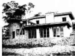
261 - The Busst House Eltham 02 - North elevation of the Busst House photographed during construction - Note the roof deck above the ground floor living room minus its balustrade which is still to be installed - Shire of Eltham Heritage Study 1992
