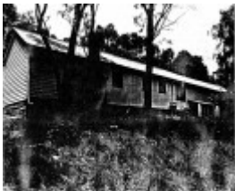
278 - Hurstbridge Railway Station Building 04 - Shire of Eltham Heritage Study 1992
