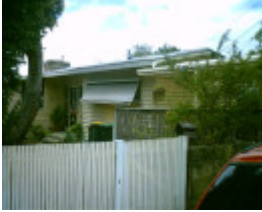
2 Lupton Street, Geelong West
