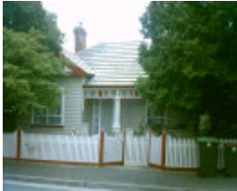
4 Lupton Street, Geelong West
