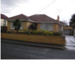
18 Clarence Street, Geelong West
