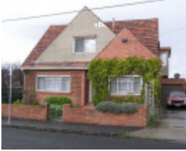
21 Clarence Street, Geelong West
