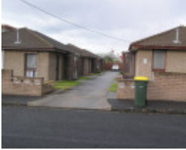
25 Clarence Street, Geelong West
