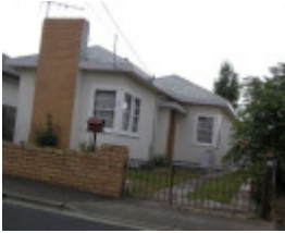
32 Clarence Street, Geelong West
