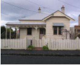
33 Clarence Street, Geelong West
