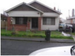
36 Clarence Street, Geelong West
