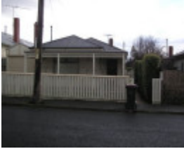
38 Clarence Street, Geelong West
