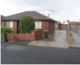
41 Clarence Street, Geelong West
