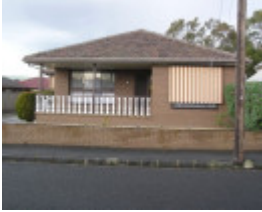
43 Clarence Street, Geelong West
