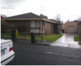
44 Clarence Street, Geelong West
