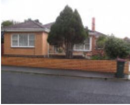
48 Clarence Street, Geelong West
