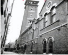
B0128 Old Fire Brigade Tower.jpg
