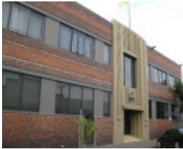
Former Charles Steele & Co. Company Factory - 9-27 Michael Street, Brunswick
