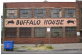
Buffalo House - 3-5 Union Street, Brunswick
