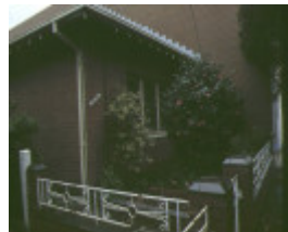
108 116 gladstone street south melbourne iron fence
