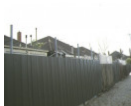
108 116 Gladstone Street South Melbourne Rear Lane View
