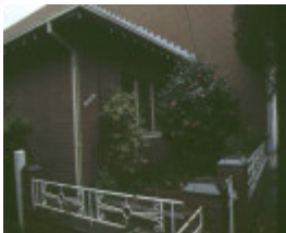
108 116 Gladstone Street South Melbourne Iron Fence
