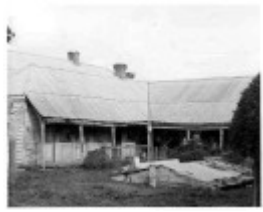
CB 05 3 - Undated photograph, State Library of Victoria Picture Collection - now demolished
