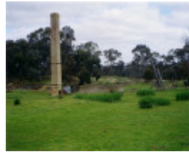
DL 10 1 - chimney used to vent a Cornish boiler for the Eucalyptus Distillery - Shire of Northern Grampians - Stage 2 Heritage Study, 2004
