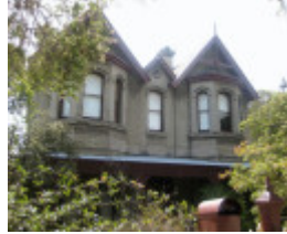
St Martin's Anglican church vicarage
