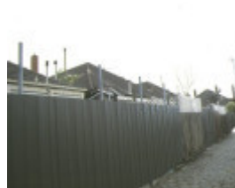
108 116 gladstone street south melbourne rear lane view
