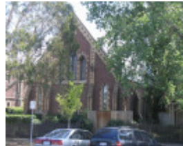
ROBERT RUSSELL HOUSE AND FORMER CONGREGATIONAL CHURCH HALL SOHE 2008
