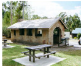
HG 03 1 - Associated Kitchen Building in the Caravan Park - Shire of Northern Grampians - Stage 2 Heritage Study, 2004
