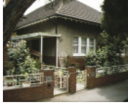
1 83 89 montague street south melbourne front gates & entrance
