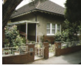
1 83 89 montague street south melbourne front gates & entrance
