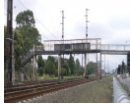
HO10 Pedestrian Footbridge 1.JPG
