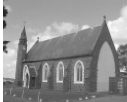
Site 036 - St Augustine's Catholic Church (2).jpg
