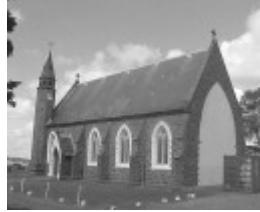
Site 036 - St Augustine's Catholic Church (2).jpg
