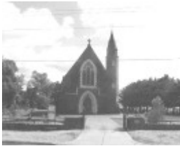
Site 036 - St Augustine's Catholic Church.jpg
