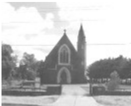
Site 036 - St Augustine's Catholic Church.jpg
