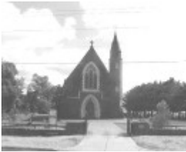
Site 036 - St Augustine's Catholic Church.jpg
