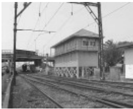
Site 026 - Sunshine railway signal box.jpg
