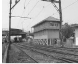
Site 026 - Sunshine railway signal box.jpg
