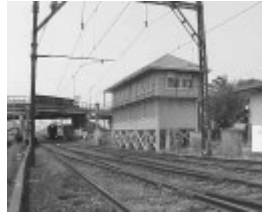
Site 026 - Sunshine railway signal box.jpg
