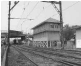
Site 026 - Sunshine railway signal box.jpg
