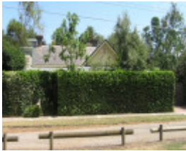
H027 Former Police Station 2.JPG
