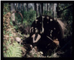
RICHARDS & SONS LOGGING WINCH SITE
