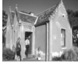
Site 017 - Overnewton gatehouse.jpg
