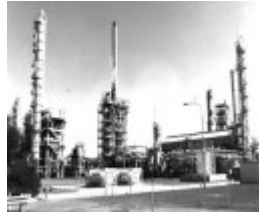
1969c - Brimbank City Council Post-contact Cultural Heritage Study 1999
