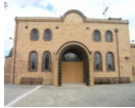
HO119 St Andrews St Greek Orthodox Church.JPG
