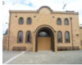
HO119 St Andrews St Greek Orthodox Church.JPG
