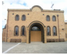
HO119 St Andrews St Greek Orthodox Church.JPG
